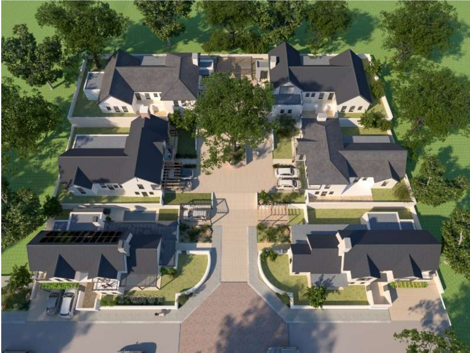
Figure 11: Typical courtyard (cul-de-sac) providing a “woonerf” environment which is safe for pedestrians
